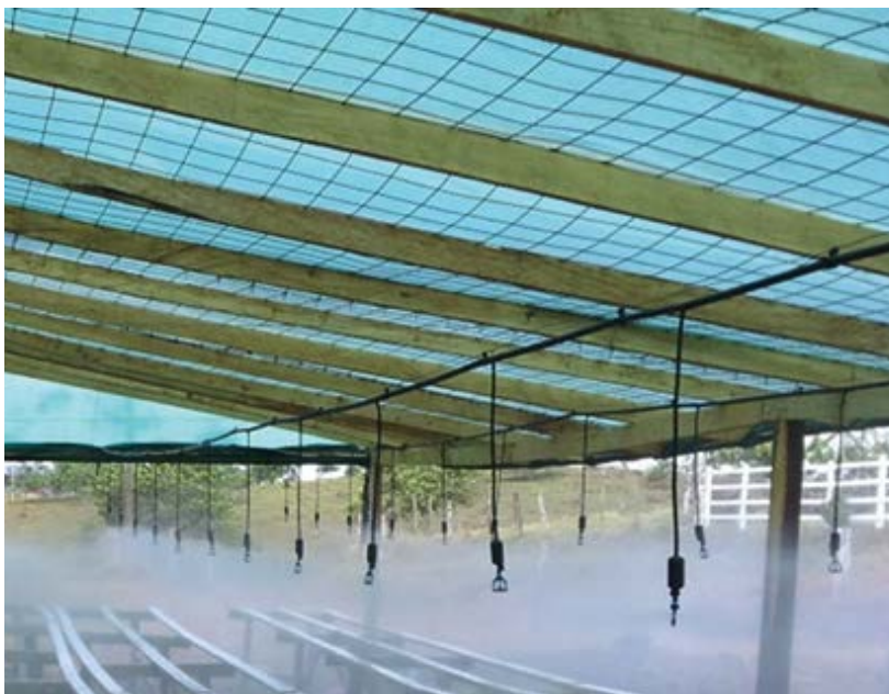
Figure 5. Wire mesh placed on the roof to support the plastic sheeting and prevent the formation of water pockets.
